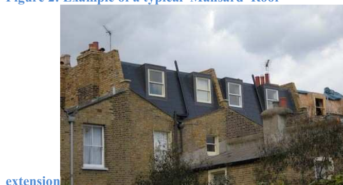
Figure 2: Example of a typical 'Mansard' Roof
